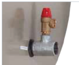
Pressure release valve
